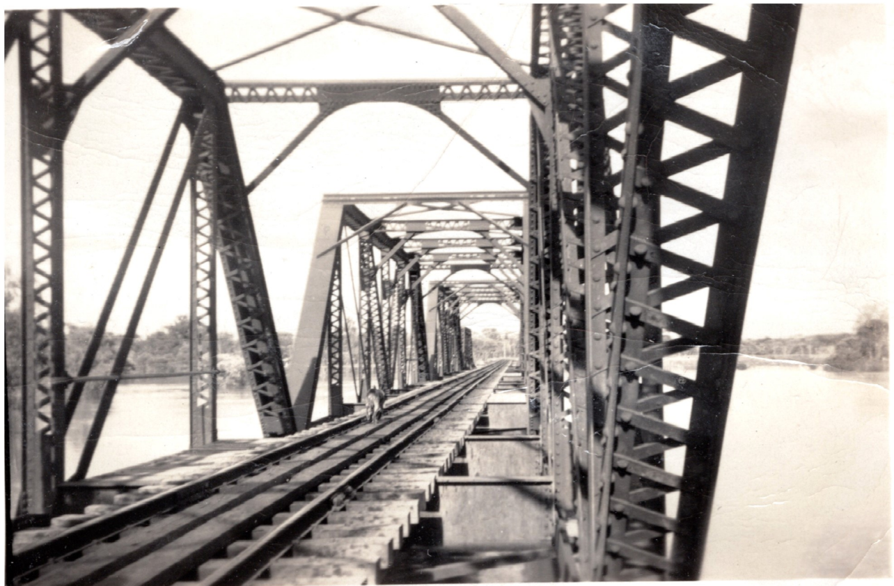
COMET STEEL RAIL BRIDGE C1953
