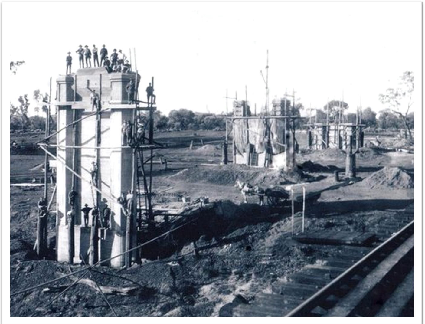
COMET STEEL BRIDGE UNDER CONSTRUCTION
