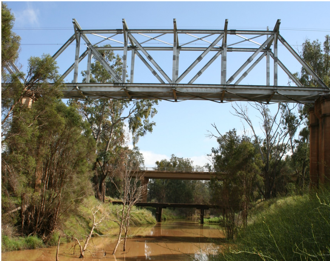
3 BRIDGES / STEEL RAIL BRIDGE, CEMENT ROAD BRIDGE OLD TIMBER ROAD BRIDGE SADLY REMOVED.
