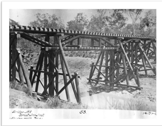
ROBERT BALLARD'S 1878 TIMBER RAIL BRIDGE
