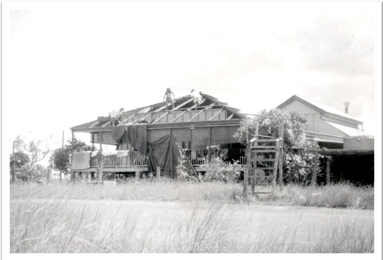
VIOLENT STORM DAMAGES CARRINGTON STORE DATE UNKNOWN
